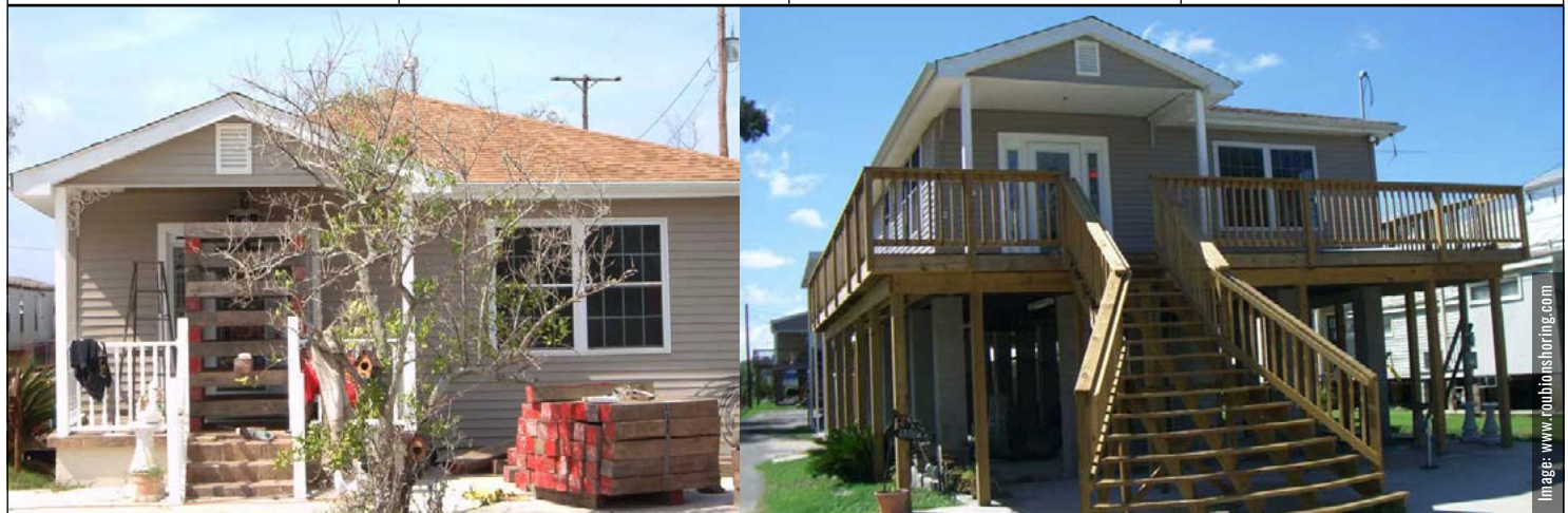
Before and After pictures of a house elevation to survive floods around New Orleans, Louisiana.
